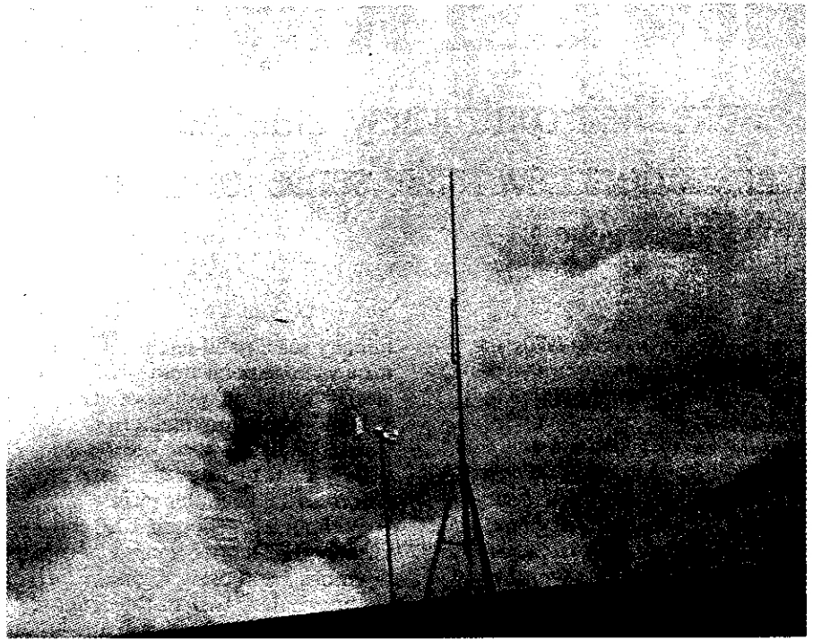
Here's one method of installing the new antenna.
